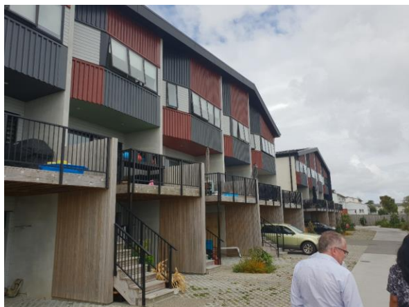
Figure 2: Exterior of side-attached homes (viewed from internal laneway).
