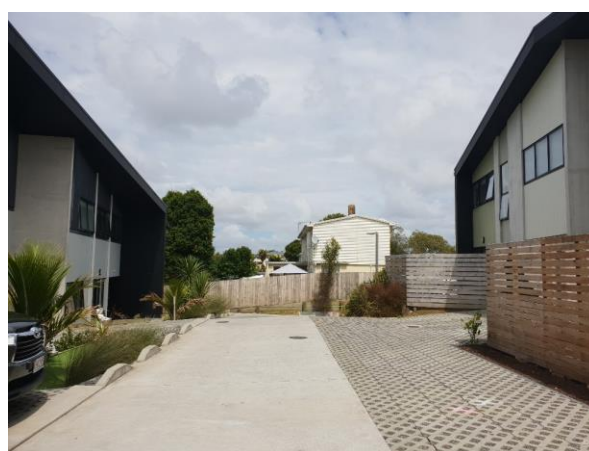
Figure 5: Shared internal laneway, including some permeable pavers to allow rainwater to soak through.
