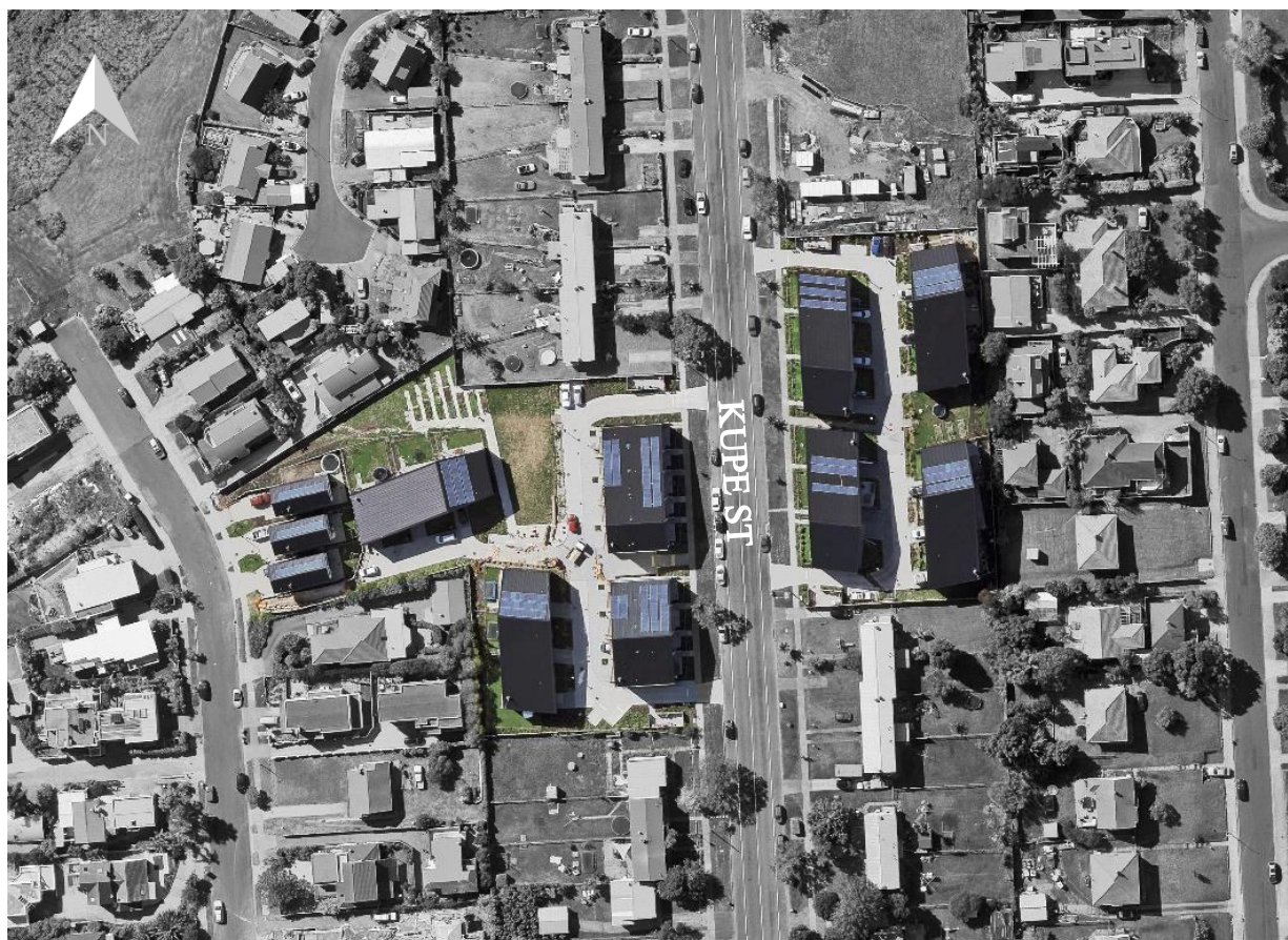
Figure 1: Kāinga Tuatahi aerial photo (development shown in colour). The development is bisected by Kupe Street down the centre, with the East Block (12 homes, in four clusters of three homes each) to the right of Kupe Street, and the West Block (18 homes) on the left.
